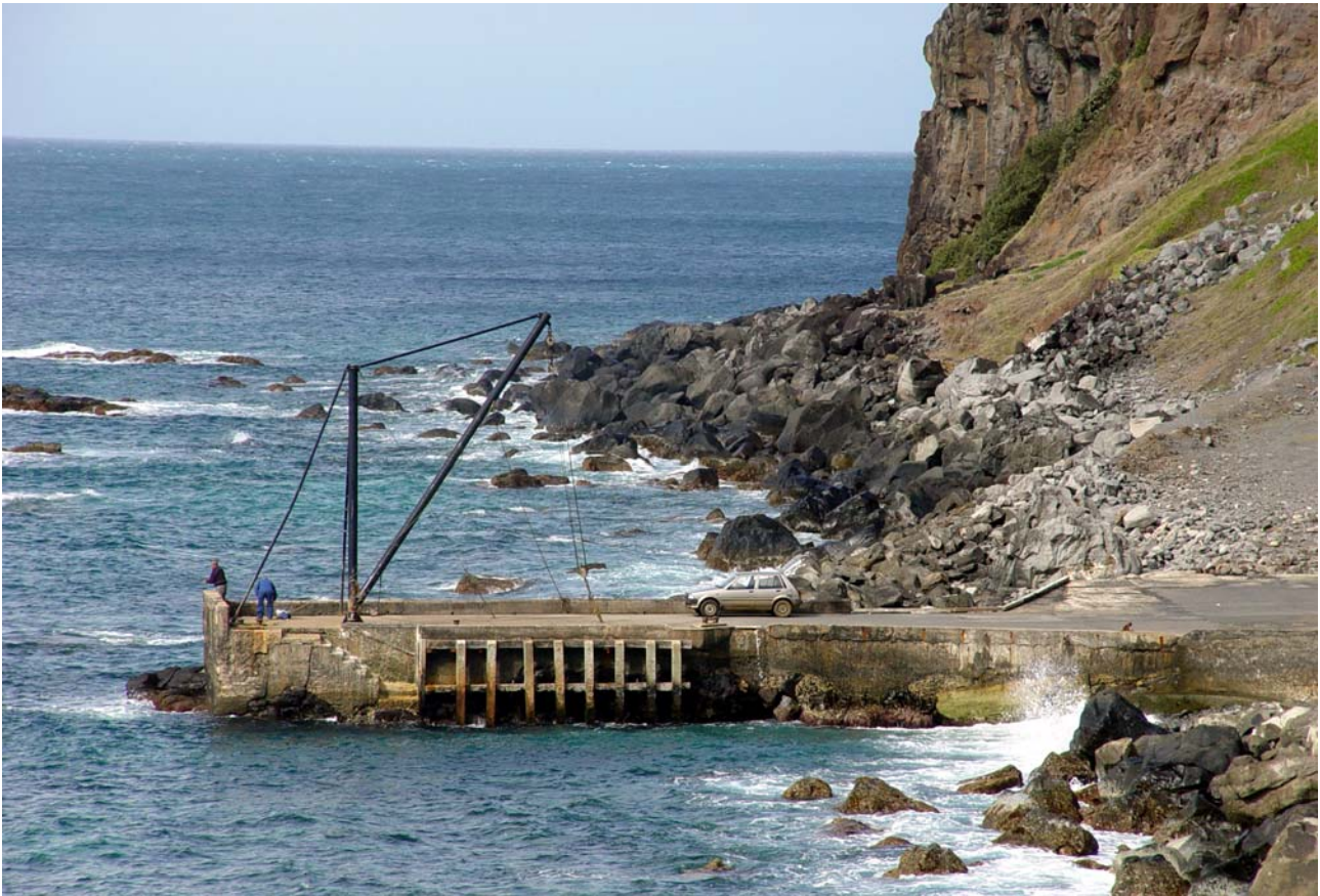
Figure 2. Jetty and crane used to deploy and retrieve boats from the water at Norfolk Island.
